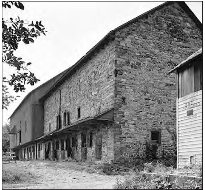
This is the original early 1940s photo of the Heller homestead barn complex, a circa 1790 English Lake District barn with a stone addition. An unusual front wall stone arch existed at the north end and a large Civil War era frame section was at the south end.
