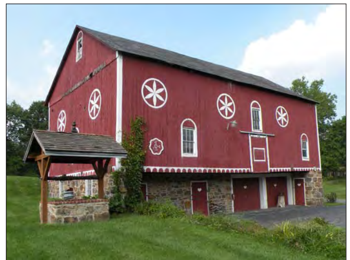
Frame Standard barn - original two-section part, circa 1860 – and one-bay addition – 1890’s
